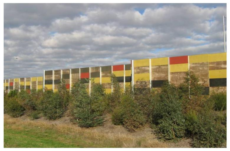
More recent plywood barriers have panels clamped inside H section steel columns.
