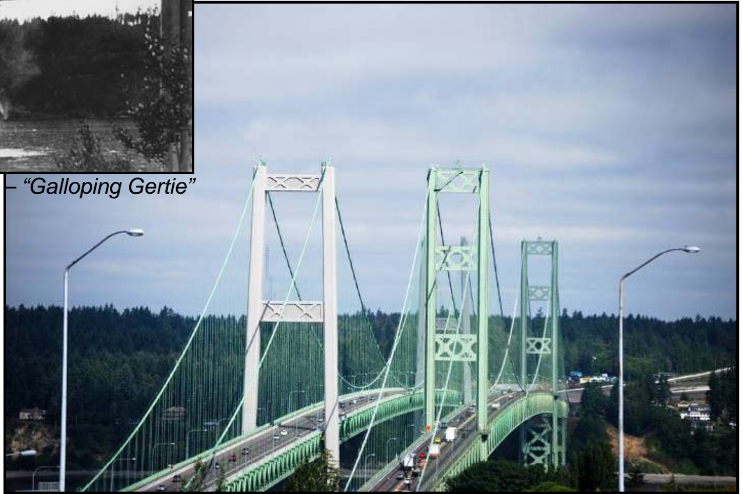
2008: New TNB (Left) finished alongside existing structure (Right)
