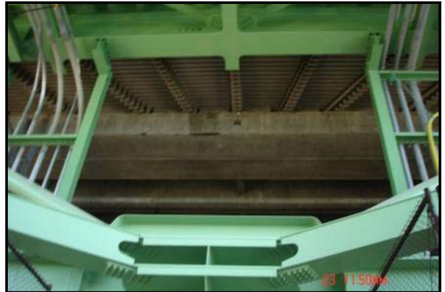
Joint installed - bottom
