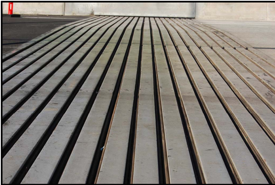
Joint installed - top
