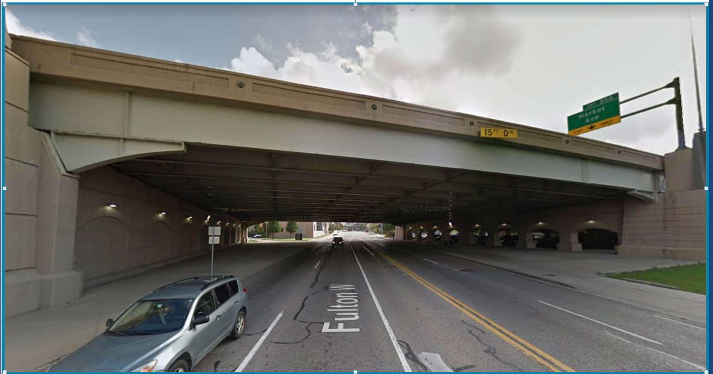
Surface street, looking East
