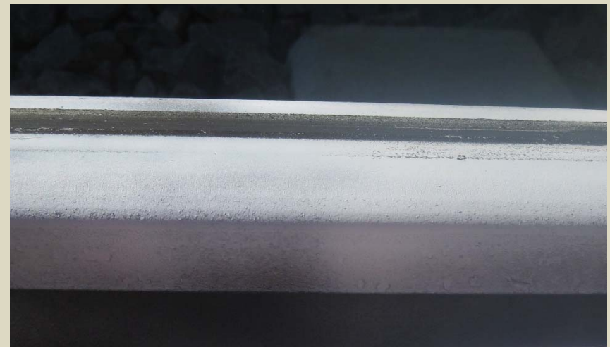
Inside (low) rail – consistent contact band
