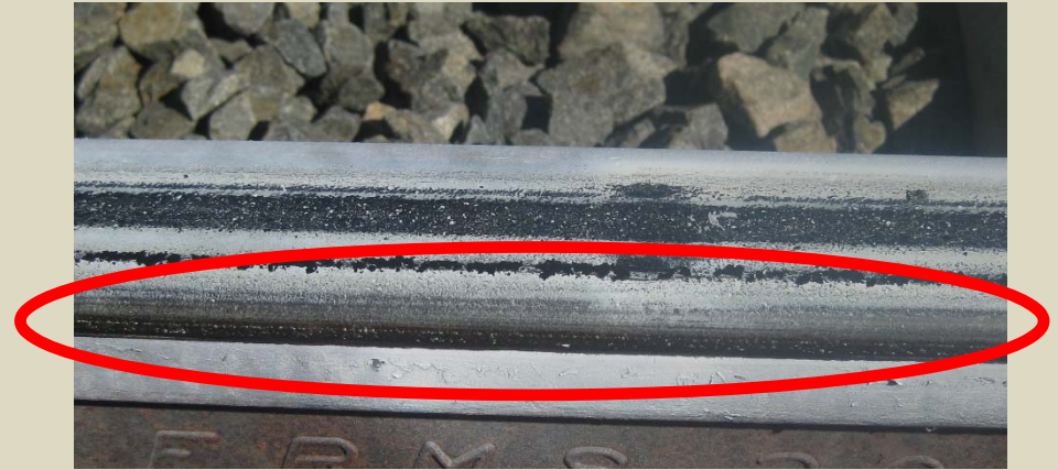
Outside (high) rail – evidence of flanging
